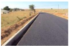
Zaaiplaas: Upgrading of public route (2.5 km) from gravel to surfaced road (using asphalt and storm water controls
